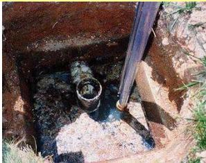
Insert six-foot long rod all the way to the bottom of the tank and let it remain for about 45-60 seconds.
