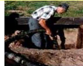
If the sludge depth measures 25 inches, or scum and sludge depth of more than one-third of the liquid depth, have a professional pump your tank.
